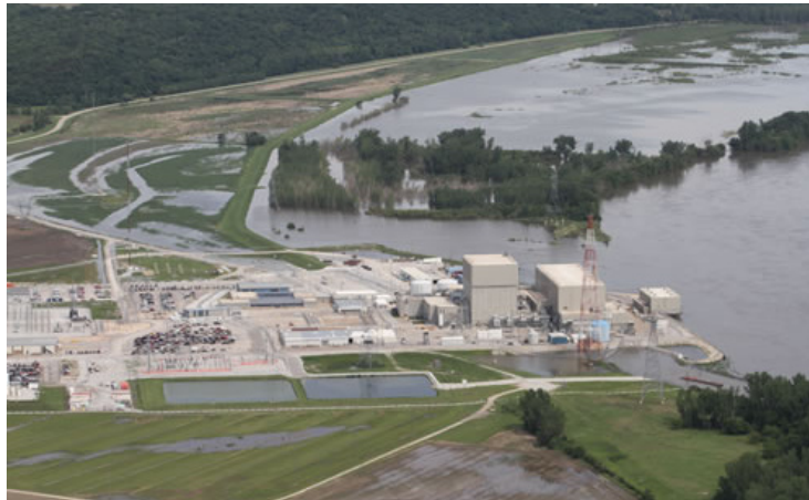
Flood waters surrounding Cooper Nuclear Station
