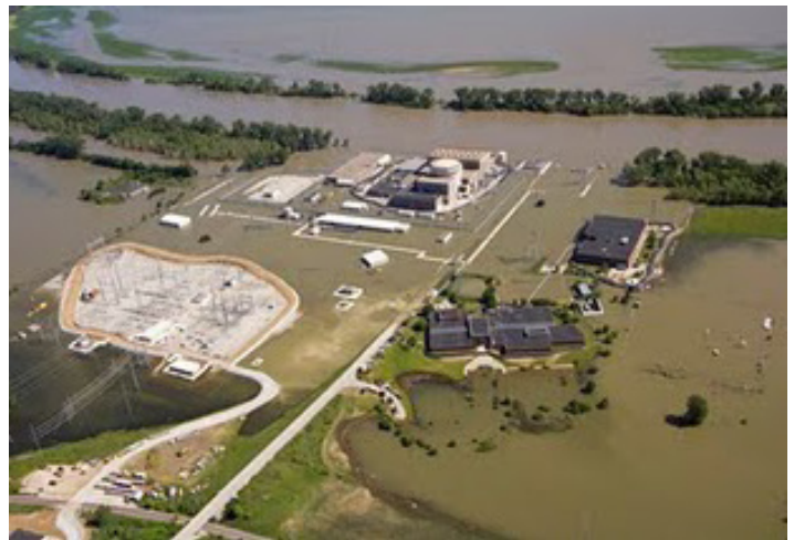
About half of the Fort Calhoun Nuclear Station plant site, about 20 miles north of Omaha, is flooded by the Missouri River.
