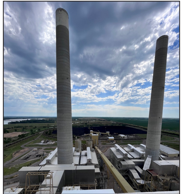
The view from the top of the east building at the Gerald Gentleman Station.
